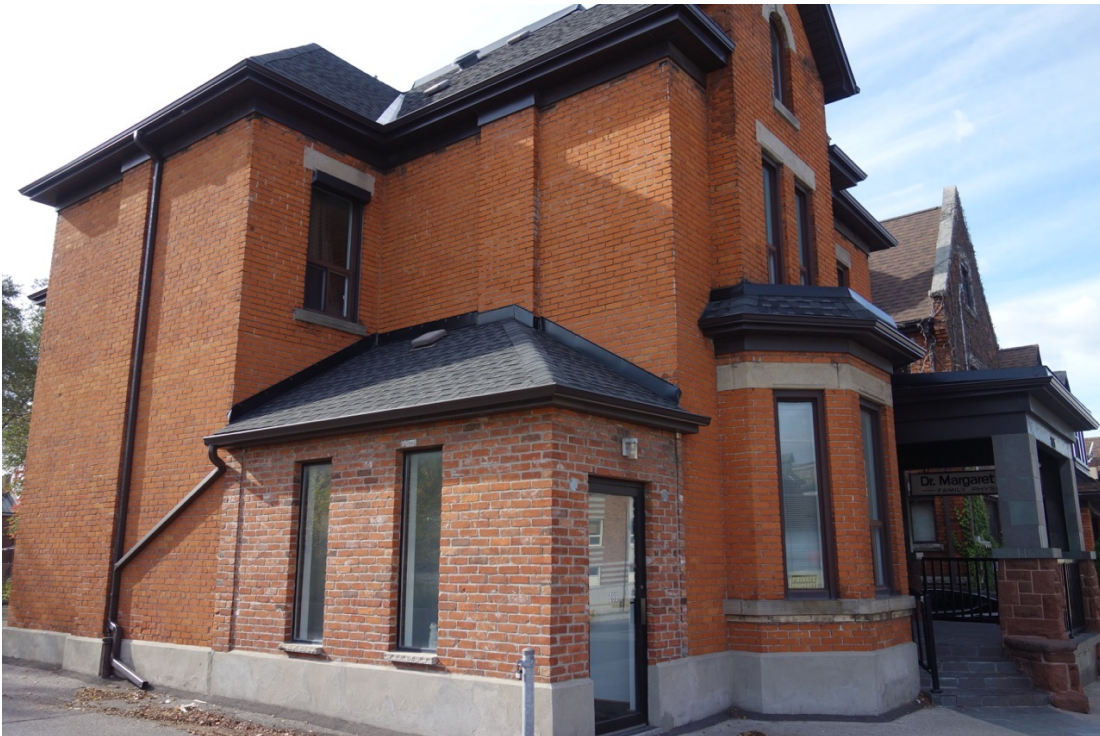
255 MAIN STREET WEST - Side façade and driveway adjacent to the development site
