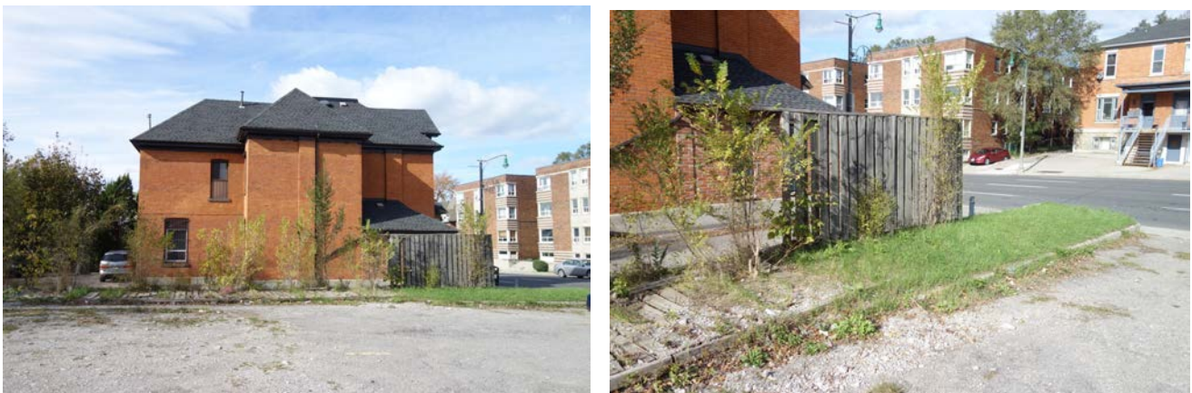
255 Main Street West – side elevation (left) – existing retaining wall and landscape strip (right)
