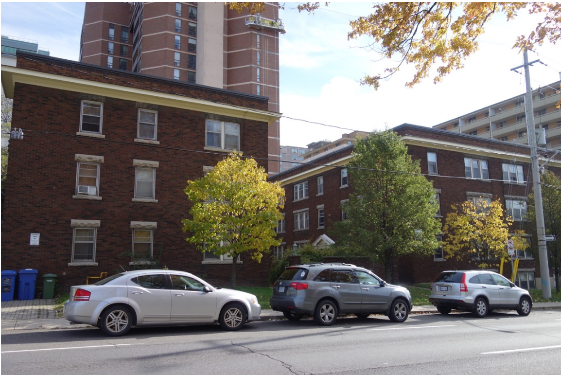
75 QUEEN STREET SOUTH – Front façade on Queen Street South
