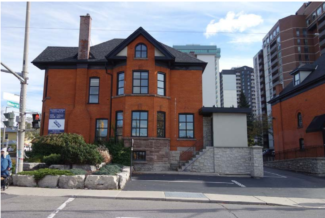
231 MAIN STREET WEST - Side façade on Queen Street South
