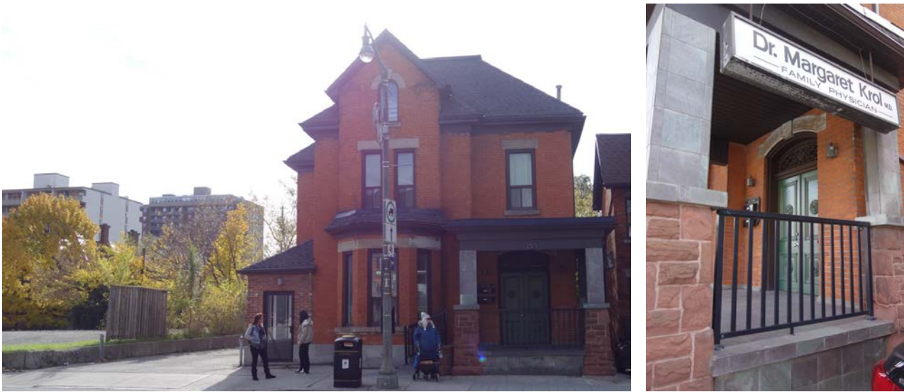
255 Main Street West – side driveway adjacent to the development site (left) – porch detail & front door (right)
