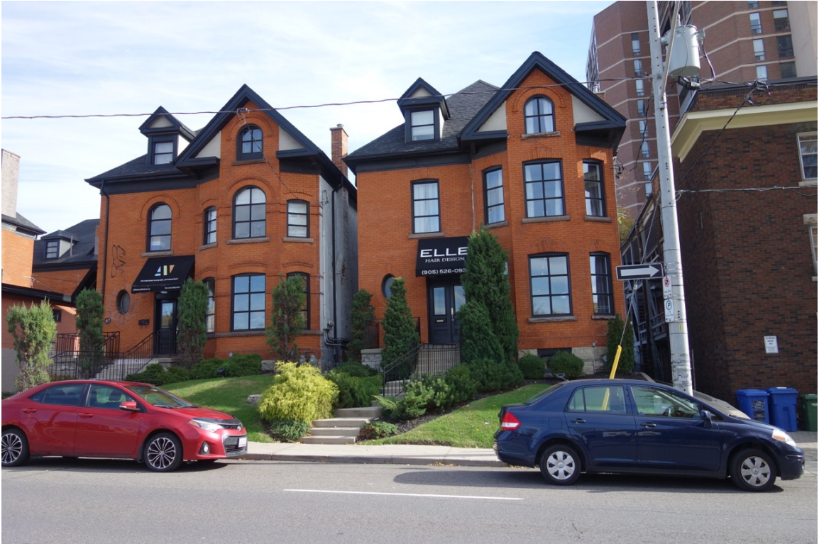
67 & 69 QUEEN STREET SOUTH – Front facades on Queen Street South
