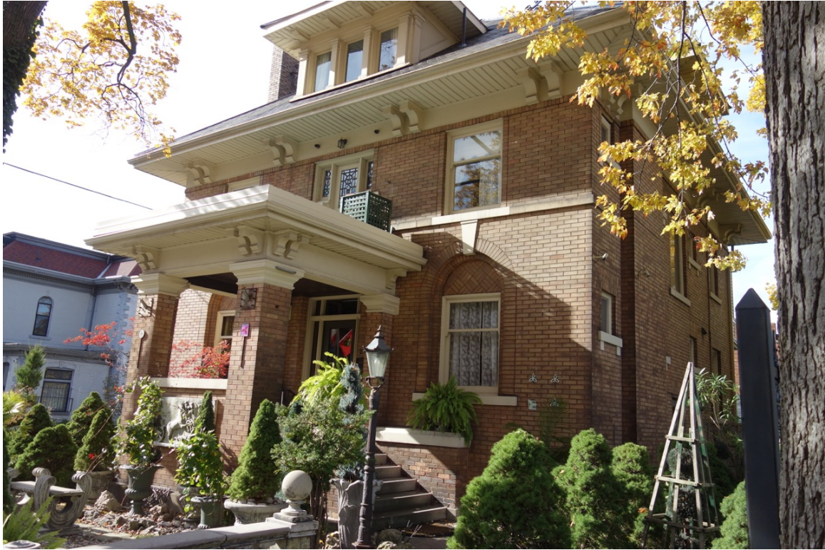
74 QUEEN STREET SOUTH – Front façade on Queen Street South
