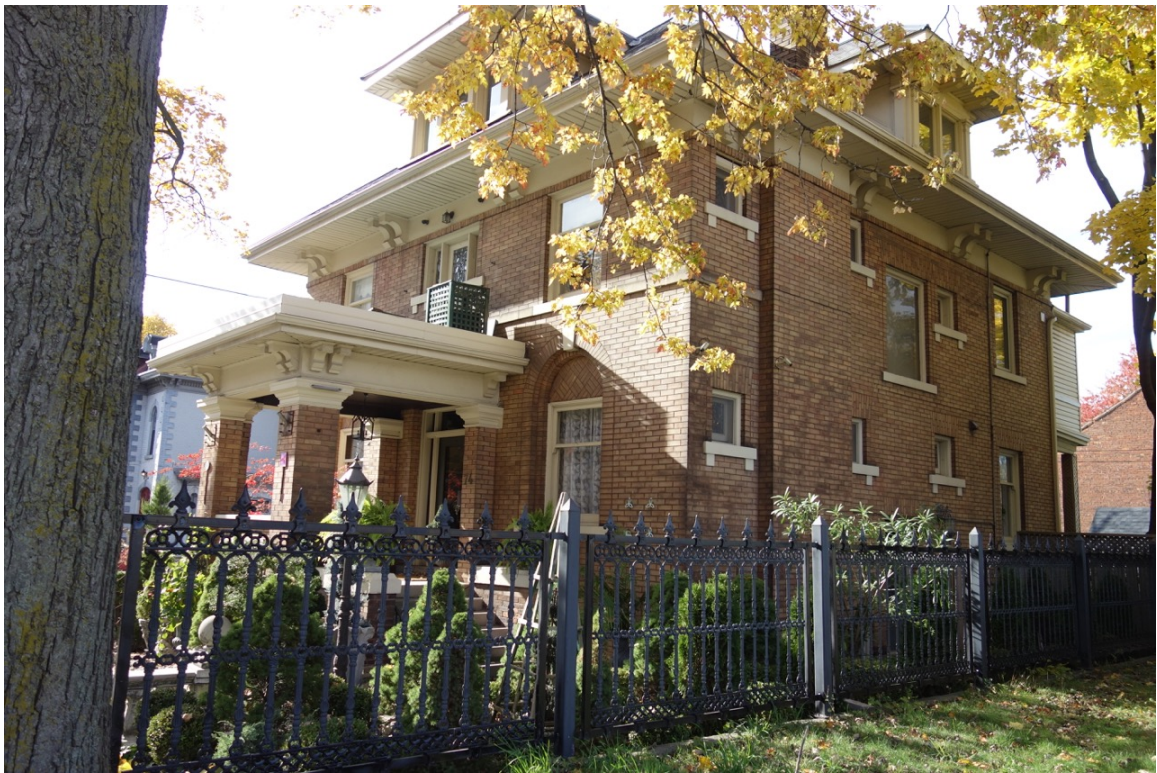
74 QUEEN STREET SOUTH - Side yard adjacent to the development site
