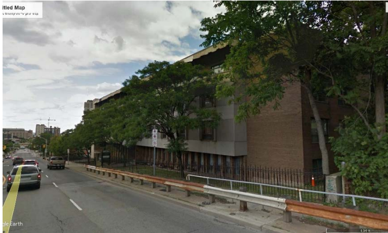
Figure 2a: Looking north at existing site
