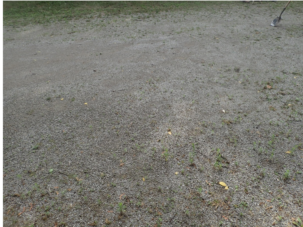
Image 5: View of disturbances associated with a gravel driveway.
