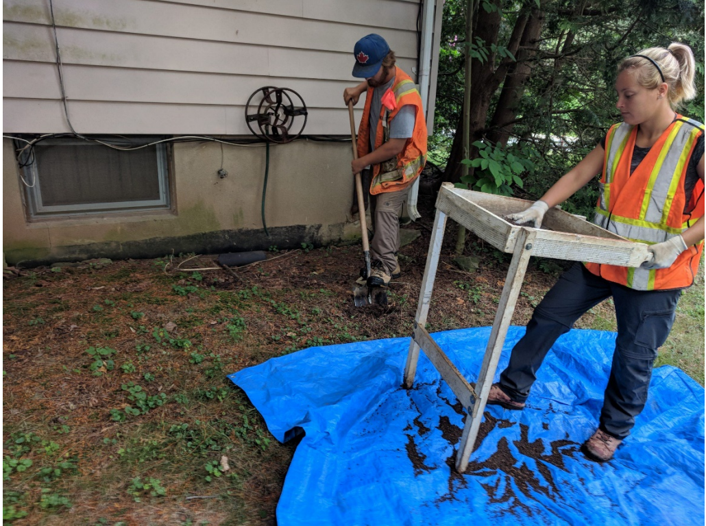
Image 9: View of test pit survey to within 1-metre of built structures.
