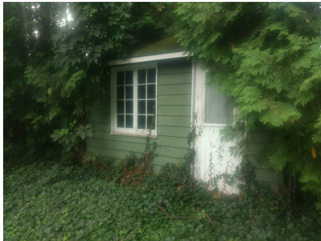
Image 7: View of disturbances associated with an outbuilding (garden shed).
