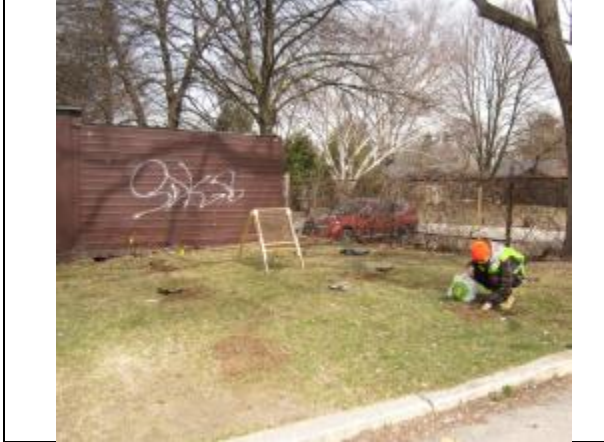
IMAGE 17 AREA OF MAIN STREET WEST SITE (NE)
