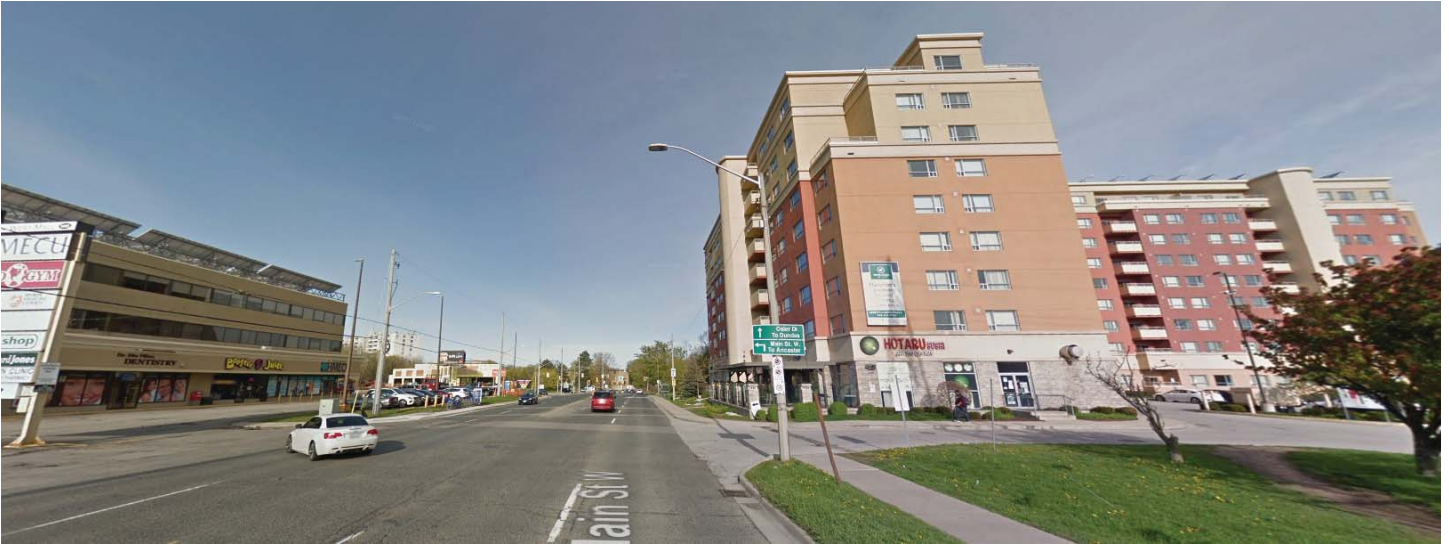
View from Main St. W. looking West Existing 9 storey student residence at 1686 Main St W.
