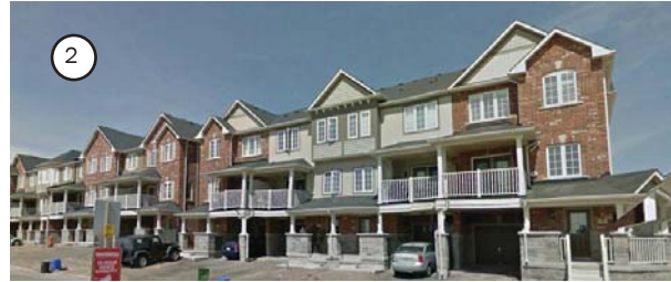
Existing Back to Back Townhouses on North Side of Nisbet Blvd.
