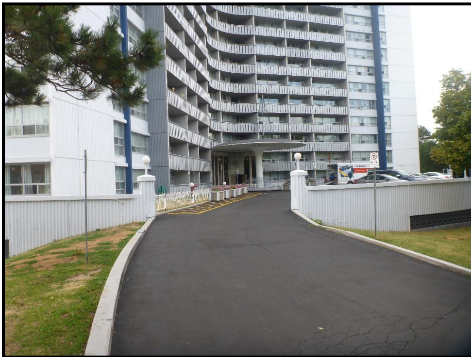
Image 2: Disturbed Lands – Apartment Building and Driveway (Facing South)
