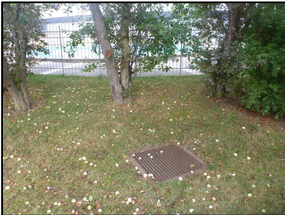
Image 6: Disturbed Lands – Sewage Infrastructure (Facing West)
