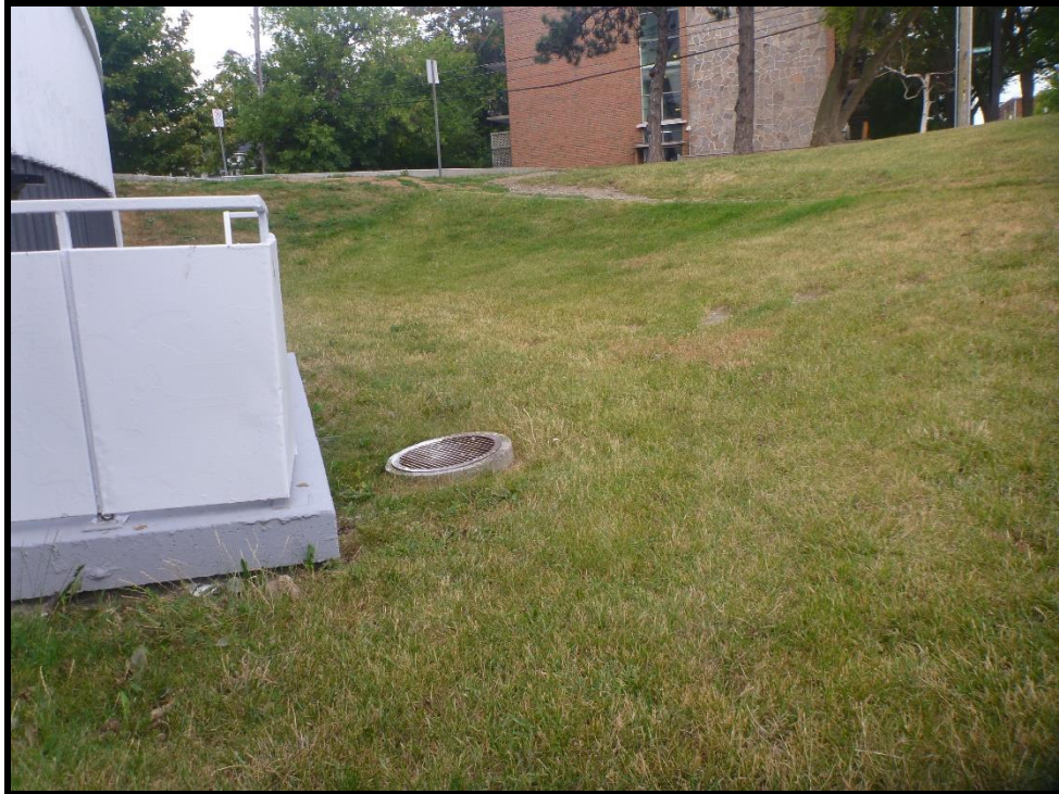
Image 7: Disturbed Lands – Sewage Infrastructure, Buildings (Facing West)
