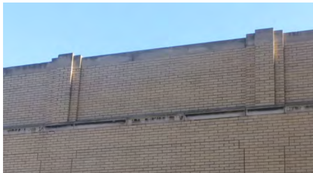
Brick and stone is generally in good condition with moderate soiling from pollution, particularly on the Hughson Street elevation.
