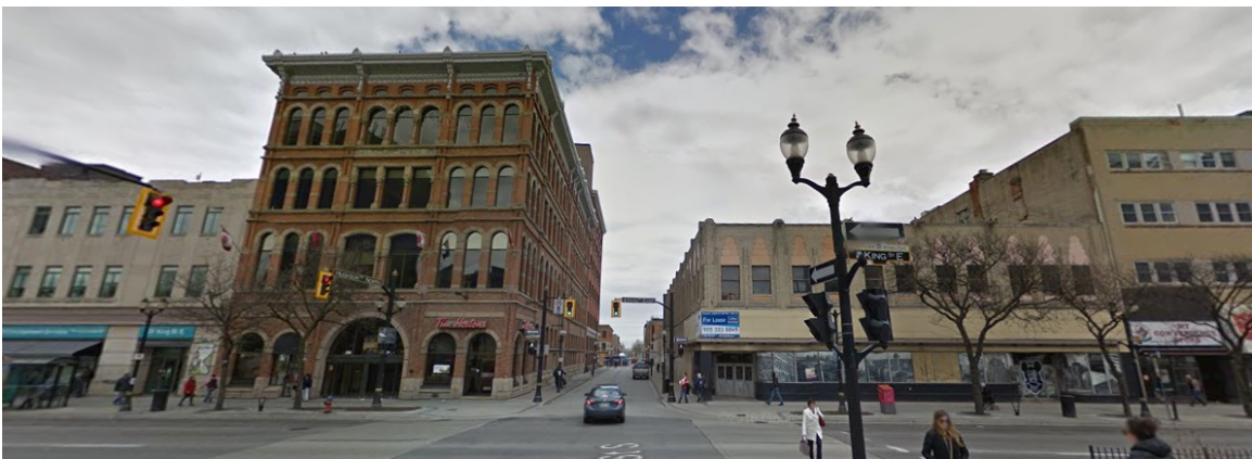
North side of King Street East.
