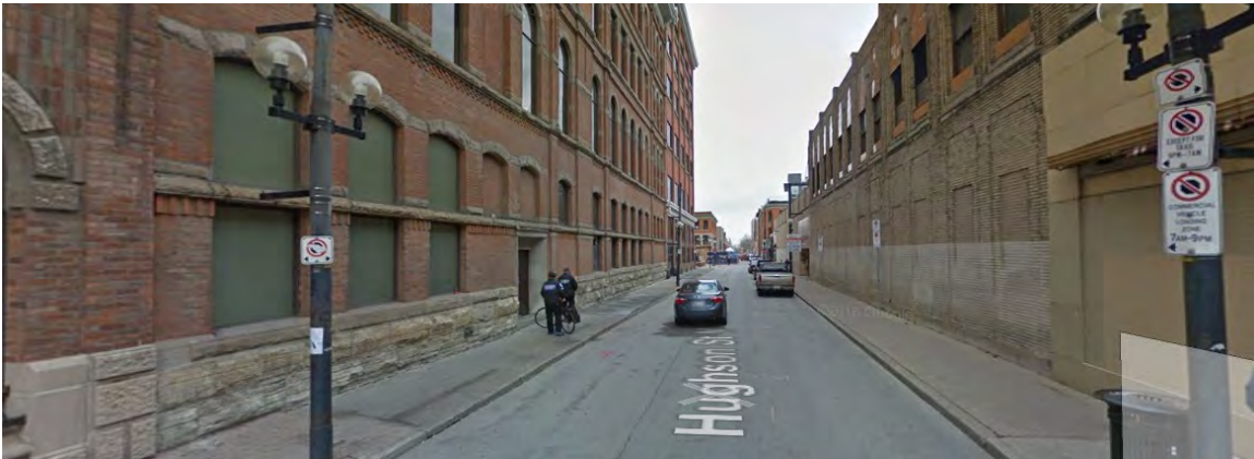
Blind windows on Hughson Street North create a tunnel like effect.
