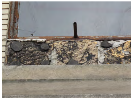
Vitrolite panels above and below the 2 nd floor window is affixed to masonry with black mastic
