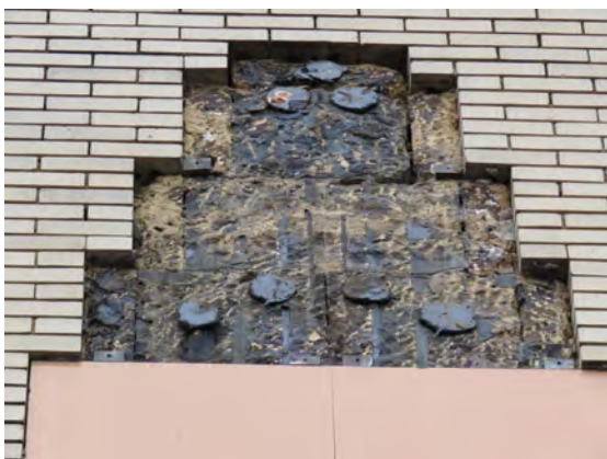
Vitrolite panels above and below the 2 nd floor window is affixed to masonry with black mastic
