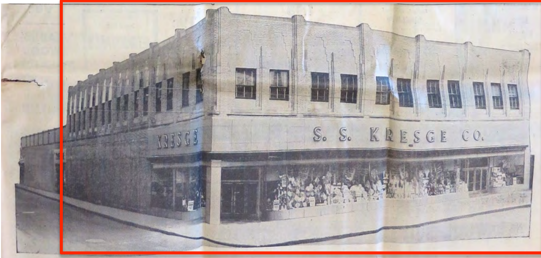
The 2-storey facades on King Street East and Hughson Street North have cultural heritage value.
