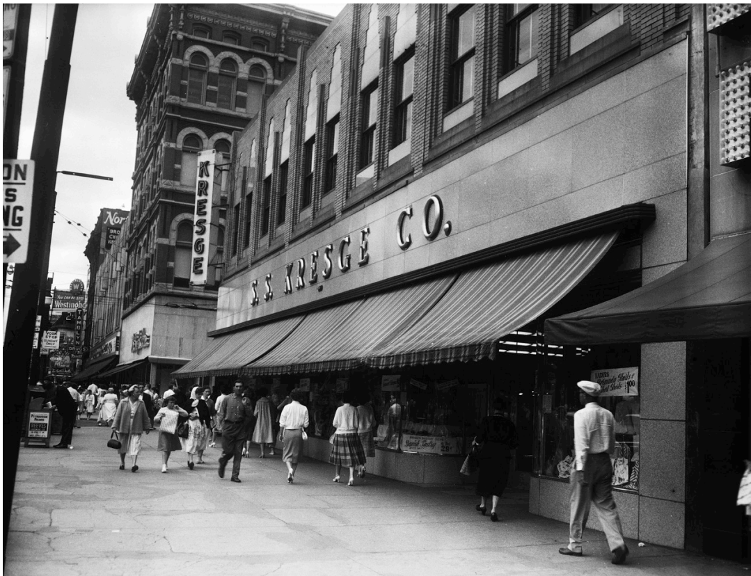
Re-modelled storefront on King Street East with new shop windows, Macotta facings, and vitrolite tiles.
