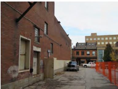
East wall of the building and view toward King William Street.
