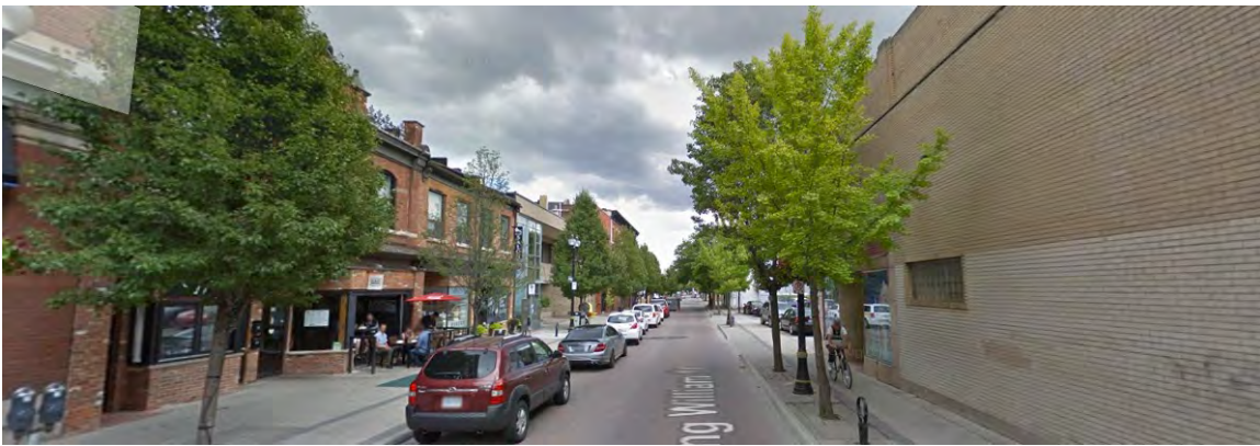
Un-articulated brick wall on King William Street.
