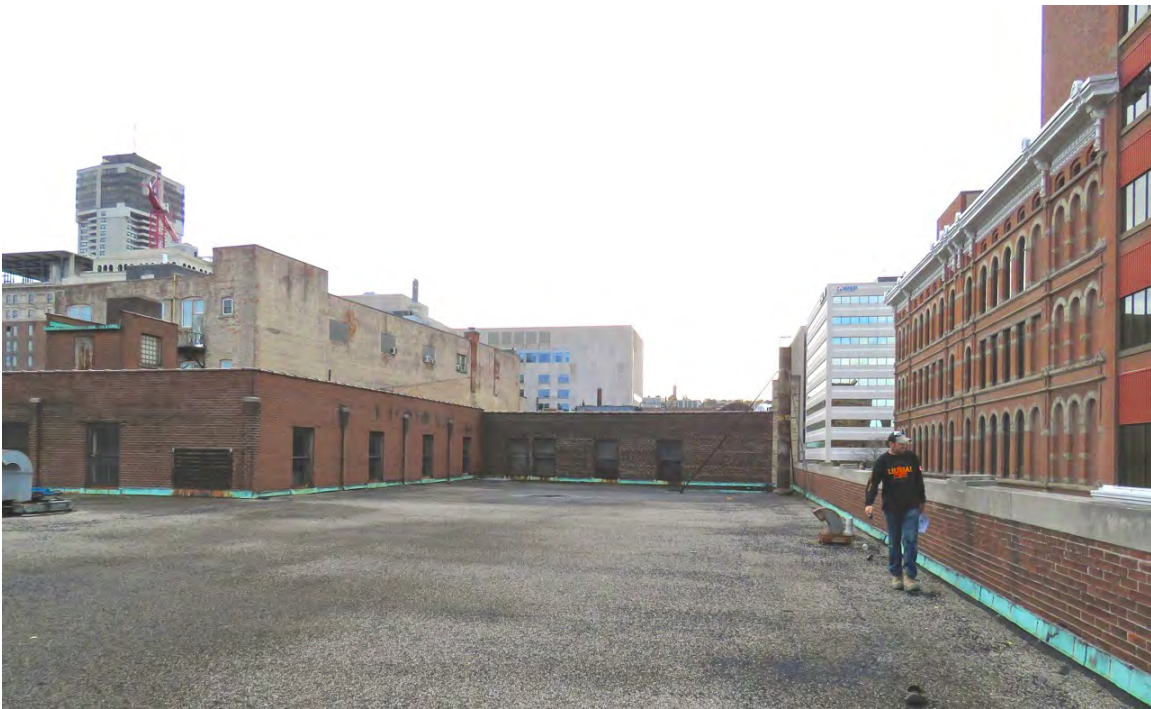
View from the roof of the one-storey rear addition looking south.
