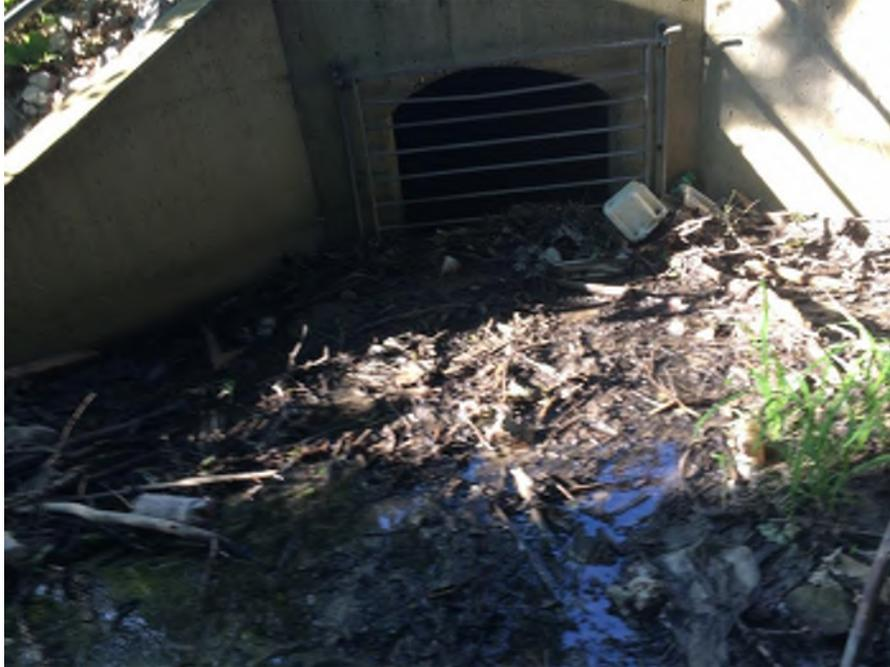
**Photo 3:** Culvert at downstream end of Study Area. No obvious flow continuing downstream of the Study Area.
