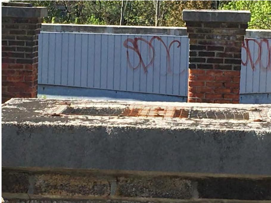
*Figure 2: Metal grating covering chimneys*
