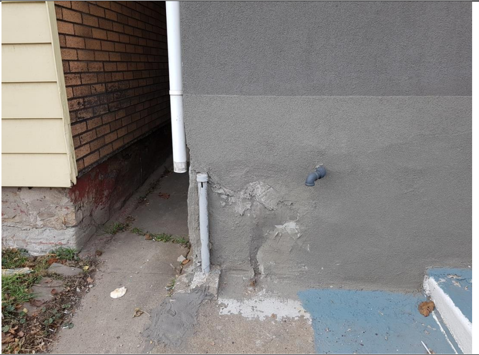
Photograph 4 Photograph depicts fill line for form AST at 255 Wellington St.N.
