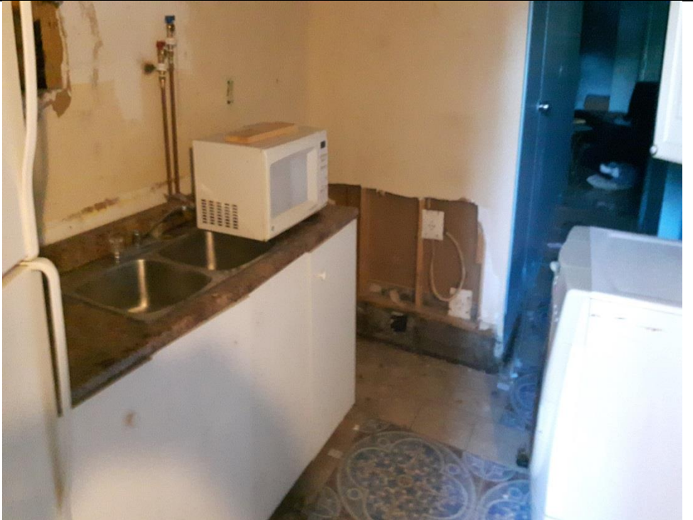
Photograph 6 Photograph depicts the interior of 257 Wellington St. N.
