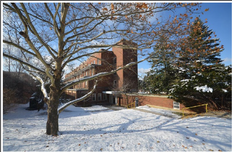
Photo 11 View from Sanatorium Drive west to Evel Building
