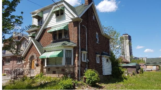
Photo 8: Disturbed House at 125 Young Street, Not Assessed, facing northwest
