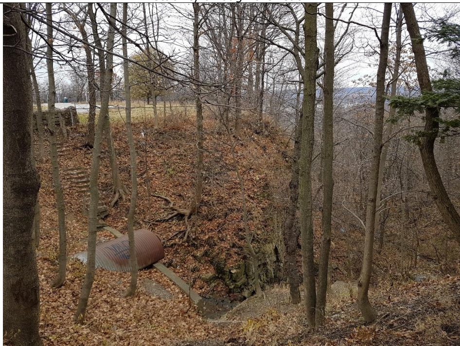
Downstream of Sanitorium Road, a rapid change in gradient was observed. The valley was confined beyond the study limits.
