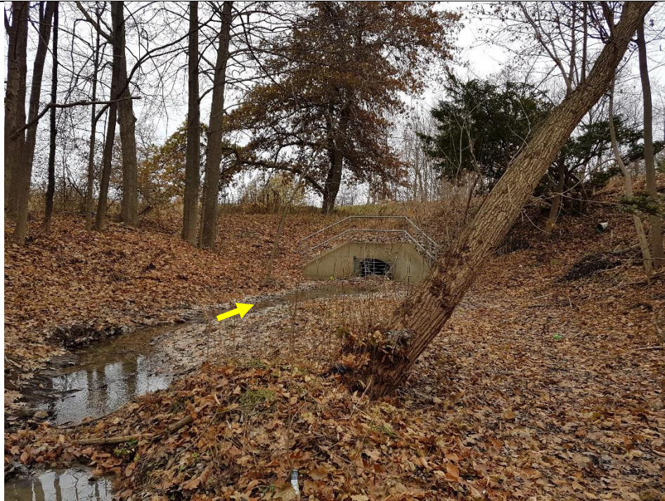
At the downstream extent of the reach, the channel entered a culvert at Sanitorium Road. Evidence of widening and degradation were the key geomorphic indicators of channel stability through the reach.
