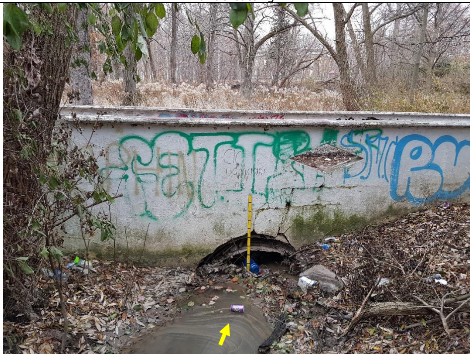
The channel flows through a corrugated steel pipe (CSP) at a pedestrian crossing mid-reach. Upstream was dominated by runs indicating poor physical instream habitat.
