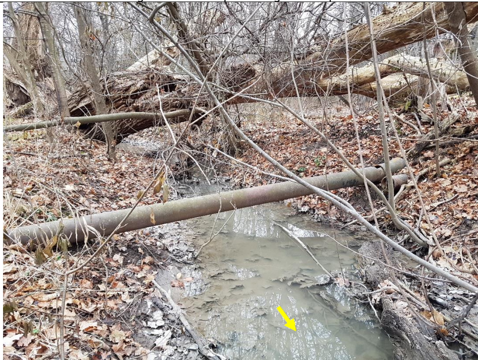
An exposed length of previously buried pipe was observed. Occurrence of large organic debris and substrate fouling was common.
