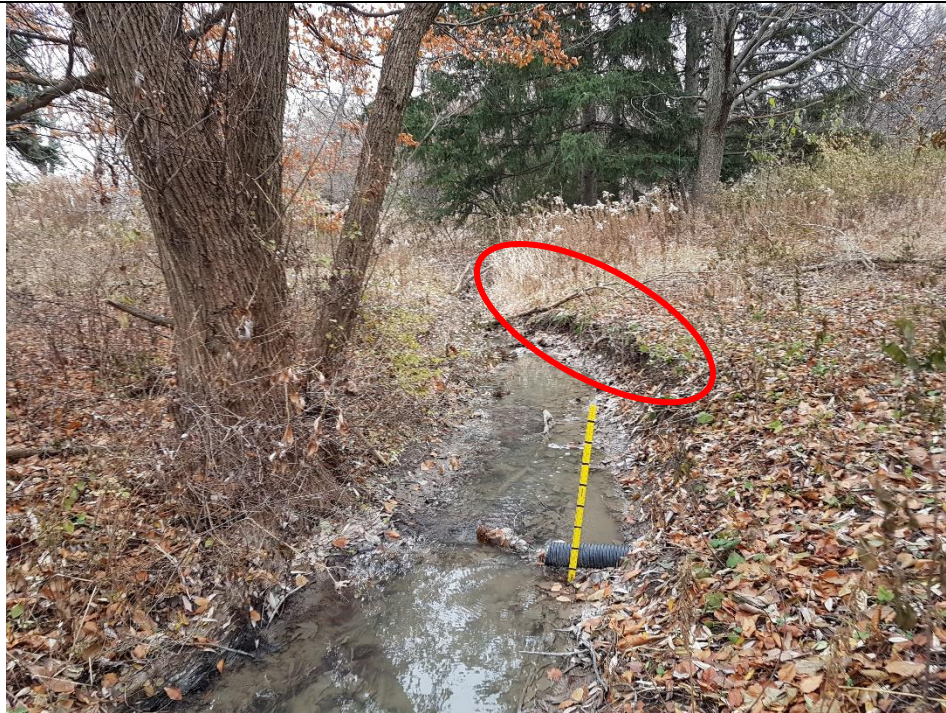
Downstream view of the channel. Bank erosion was present through 60 to 100% of the subject reach and was observed through scouring of the channel banks (circled) and undercutting.
