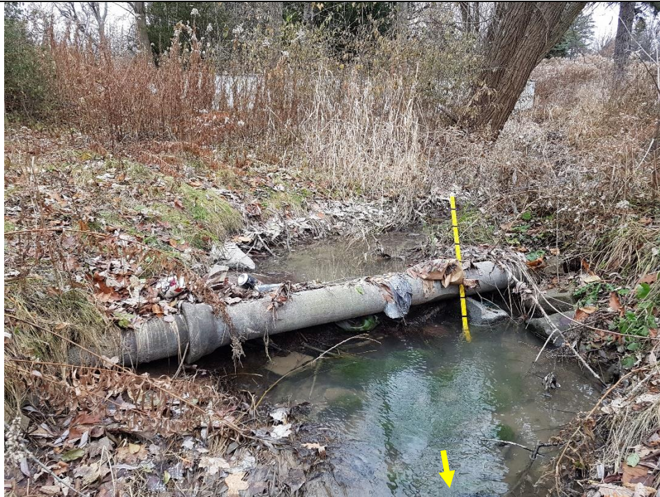
An additional length of exposed sanitary/storm sewer/pipeline was observed downstream of the pedestrian crossing providing further evidence of degradation.
