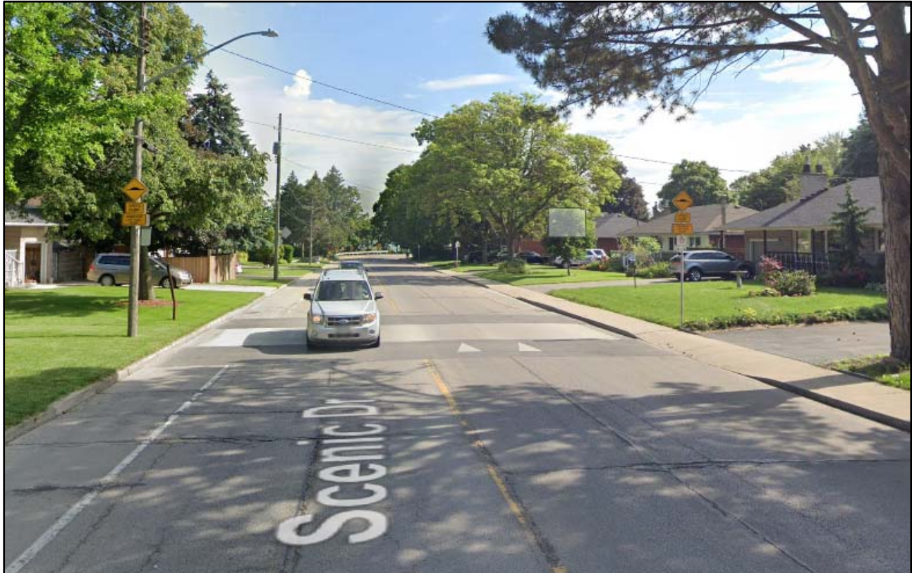
Figure 4 – Existing Speed Hump on Scenic Drive
