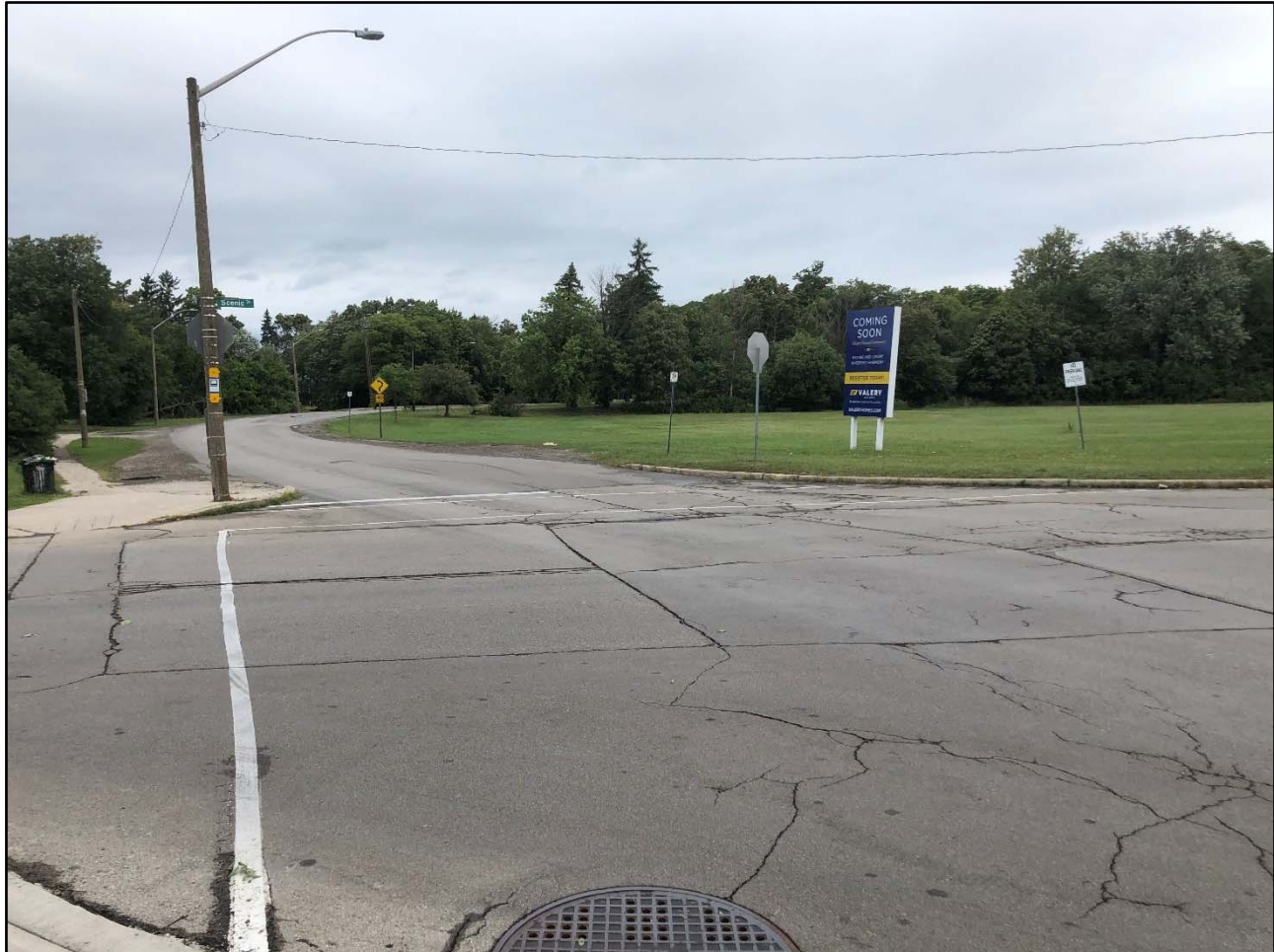
Figure 3 – Sanatorium Road Looking North
