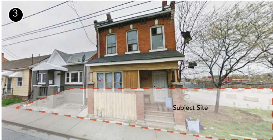
Partial view of the subject site: facing west are the two previously existing buildings located on the south corner of the subject site, now demolished.
