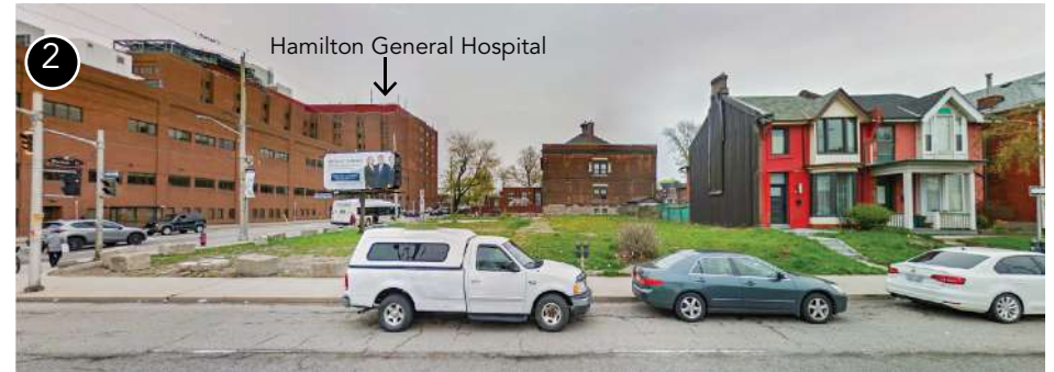
Wellington St N looking west, across the street from the subject site. On Wellington there are several 1-2 1/2 storey single family homes with approximately 6 m setbacks. Hamilton General Hospital on Barton St can be seen beyond is 4 to 8 storeys tall.
