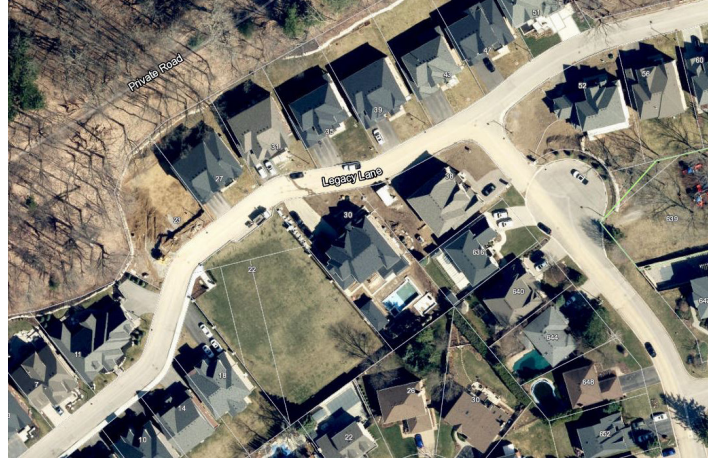
Ancaster Legacy Project Private Condominium Road Aerial View
