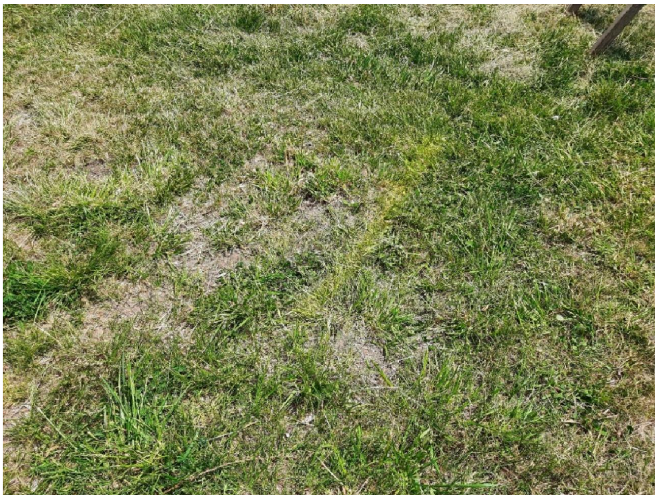
Image 8: Faint yellow paint line marking buried gas main in southwest portion.
