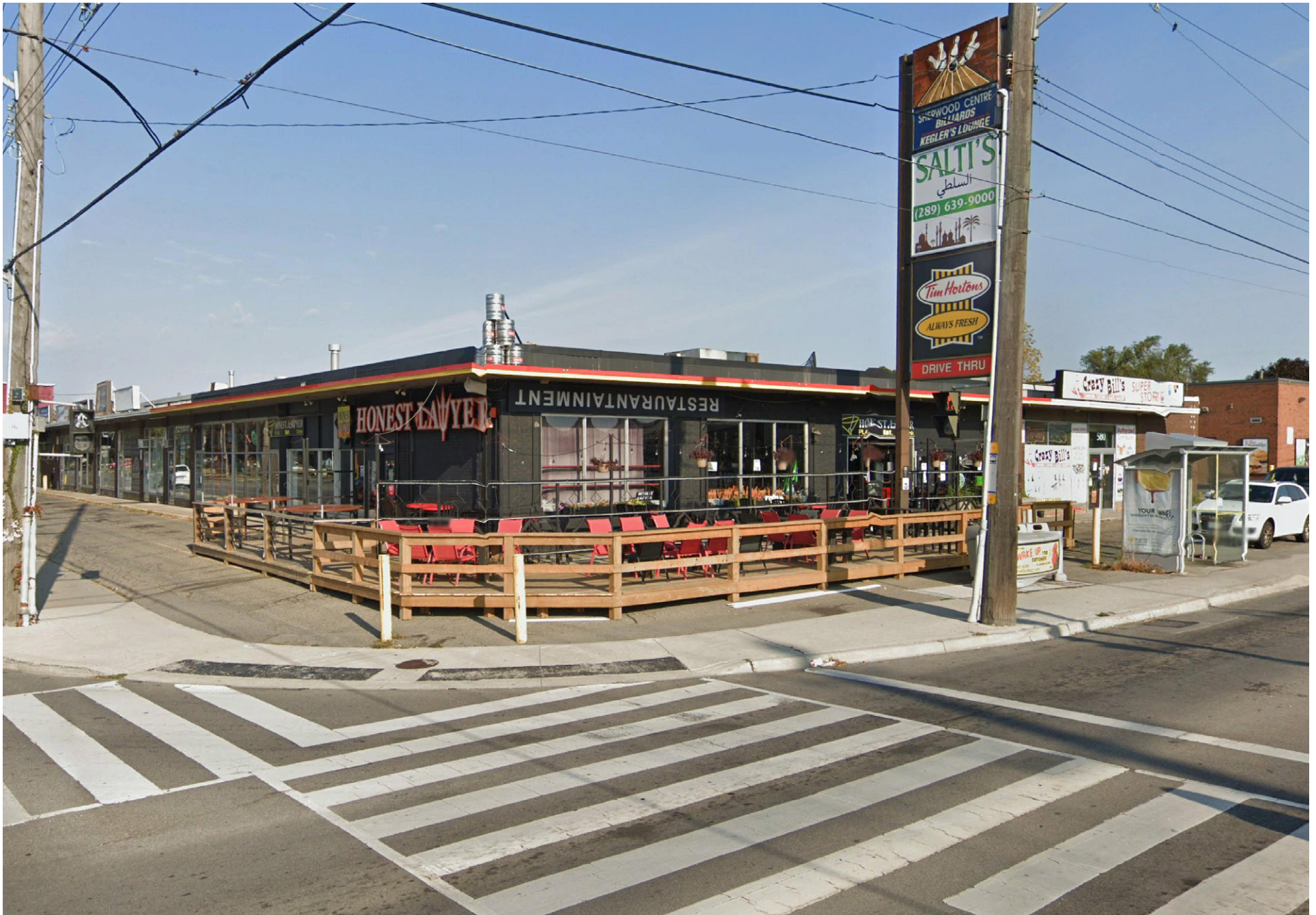
View of existing building (the "Site") looking from Fennell Avenue East and Upper Ottawa Street intersection.
