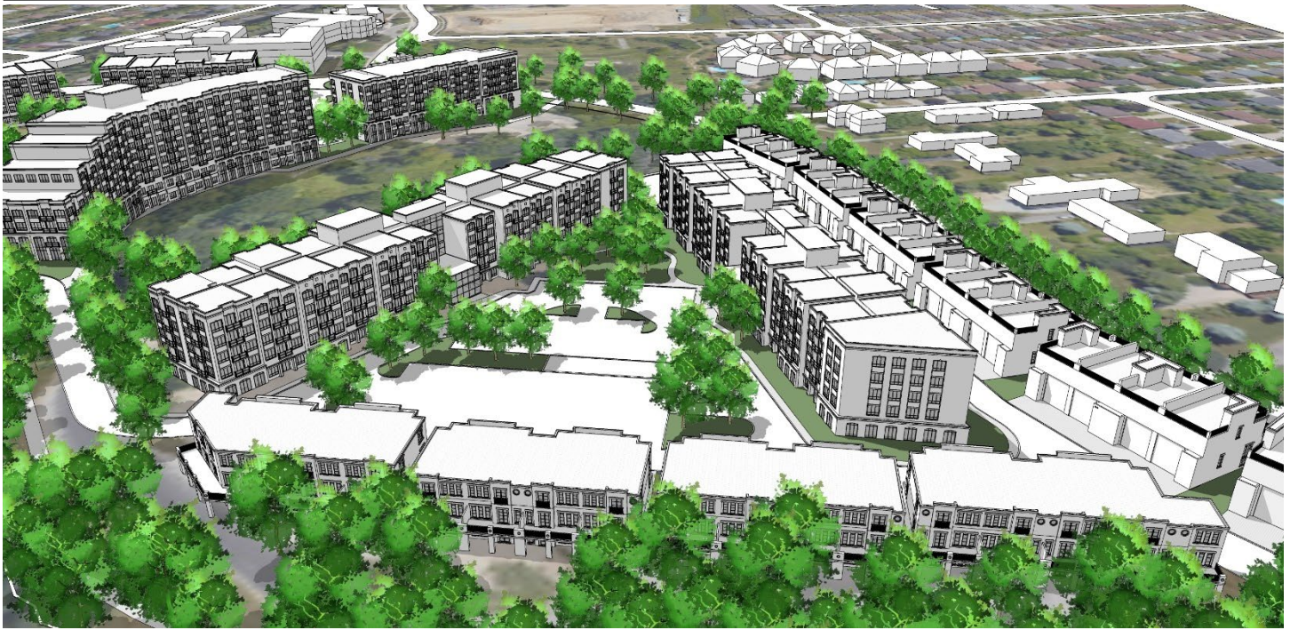
View to southeast with the landscaped garden court framed by building D and E wings. Brow Park and Trail in the foreground
