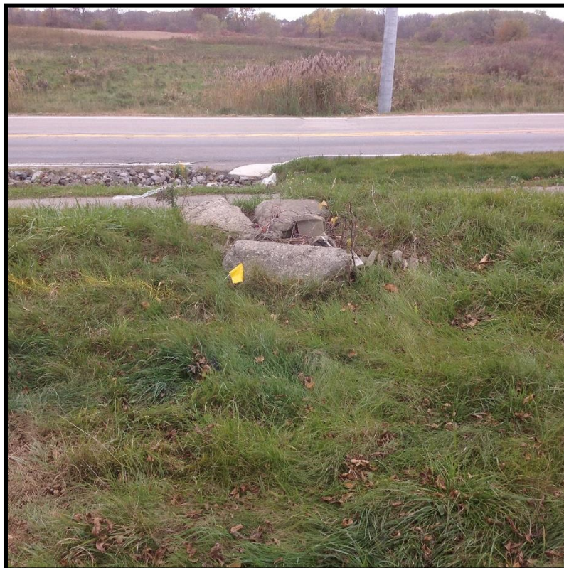
Image 6: Environs, concrete rubble facing west
