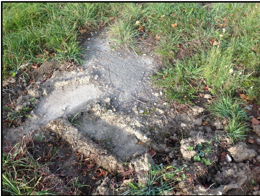
Image 4: Environs, concrete visible on surface facing west
