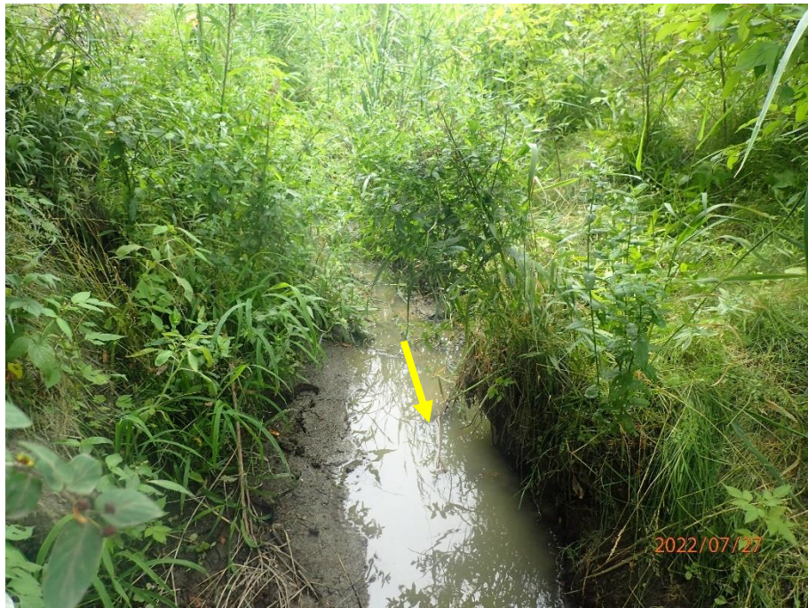
The channel bed was wetted, but flows were minimal and imperceptible during the time of assessment.
