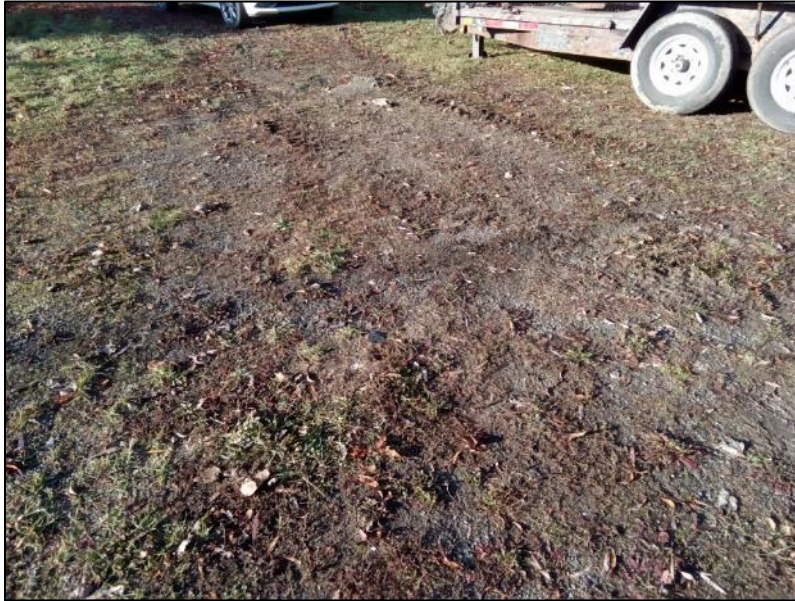
Image 1: View of the compacted gravel driveway.
