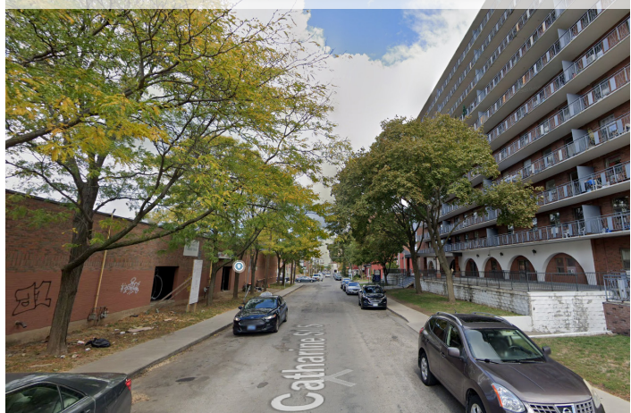
View towards the north on Catharine Street South
