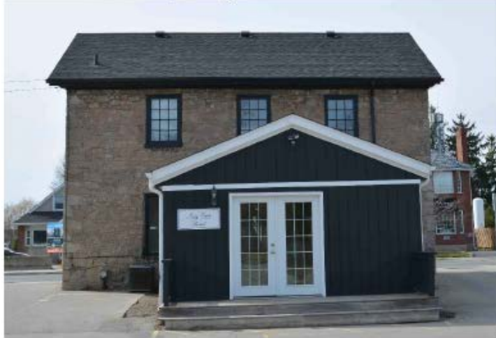
Figure 6: West End of South Wall
