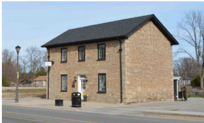
Figure 1: View from Wilson Street East – South-West Corner
