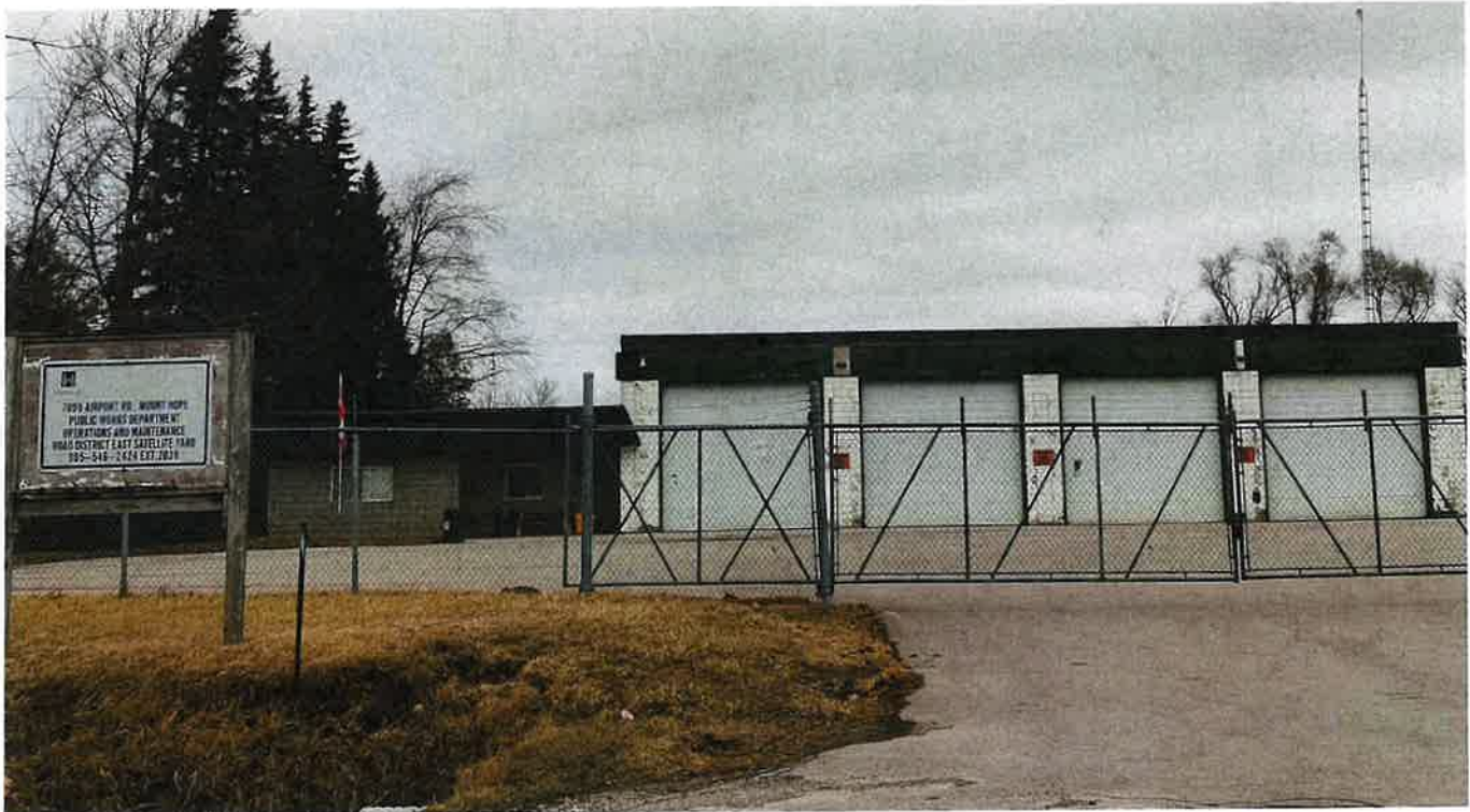
View of City of Hamilton operation and maintenance yard adjacent to the northeast of the subject site (looking north)
