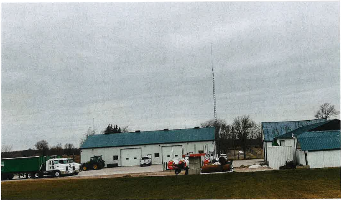
General view of northern barn in the north-eastern portion of the subject site (looking north)
