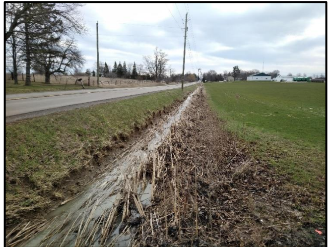
Photograph 4. Downstream View of DF2 Taken During Round 1
