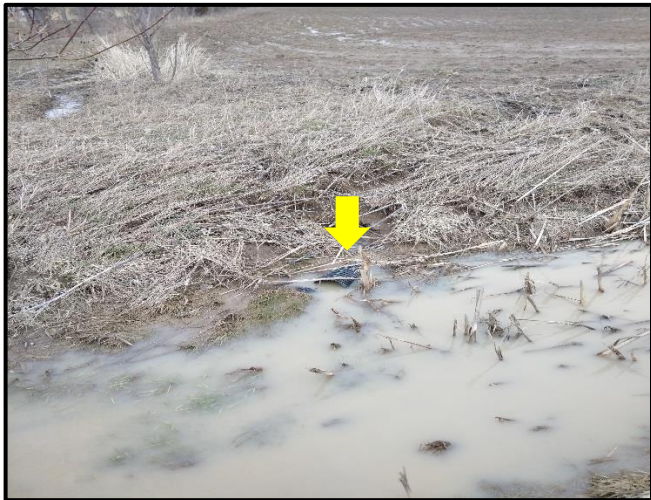
Photograph 24. Upstream View of Tile Drain Outlet (arrow) Associated with DF7 Taken During Round 1. View: N Date Taken: April 6, 2023 Site: Parcel 10
